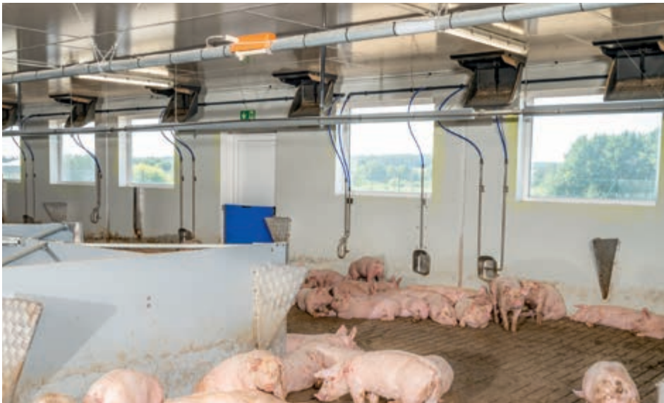
CL 1540: wide open inlet flap in the summer
