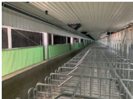
Service centre with roller curtain and RainMaker with CrossTunnel ventilation
