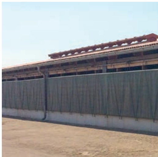
Roller curtain opening from the top to the bottom using the EWA actuator
