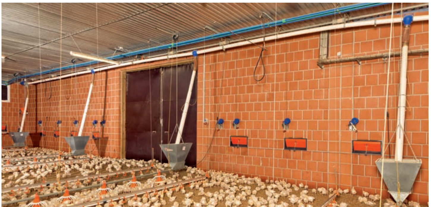
Cable winches for optimum height adjustment of the drinker lines in relation to the birds' age
