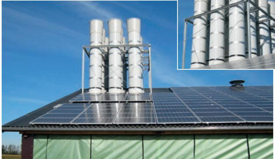
As an alternative to the extension of individual chimneys until they have reached the required height, a separate exhaust air tower can be erected at one gable end. This solution is more
