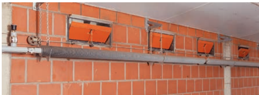
Aluminium fin heater: ideal in combination with CL 1200 fresh air inlets
