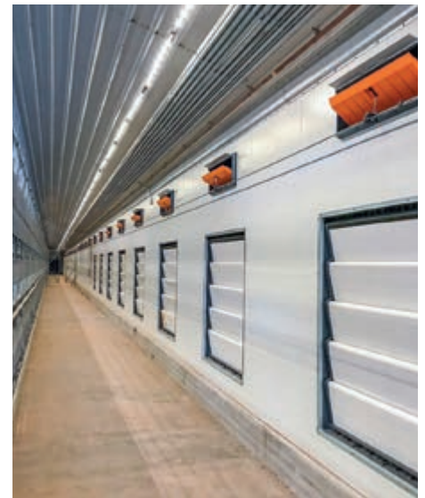
Aviary house with CombiTunnel ventilation, equipped with CL-3-1911/F flange inlets and MVT shutters
