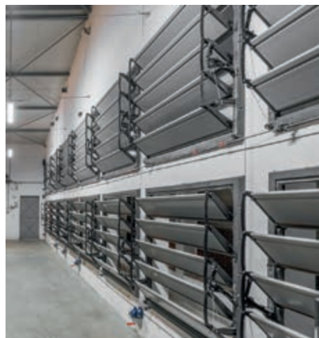
MultiVent 17 M in the gable wall for tunnel ventilation
