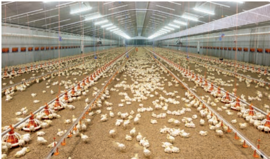
Typical broiler house in Northern Europe with fresh air supply through CL-3-1911/F flange inlets
