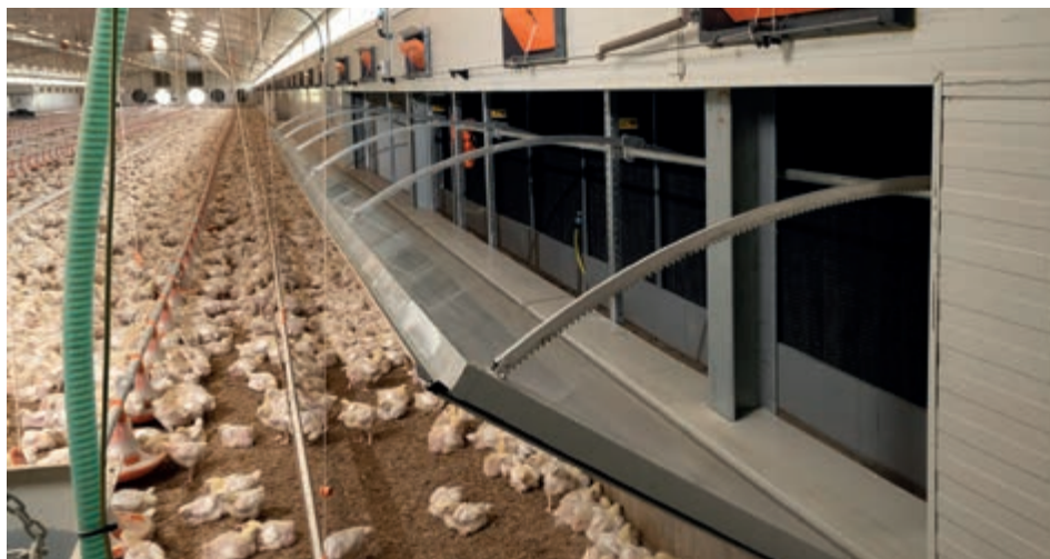
Broiler house with tunnel door, opening into the building
