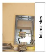
4. The Start/Stop/Emergency Stop control panel. This panel is used to start the process of removing the birds. One such panel is required per farm.
