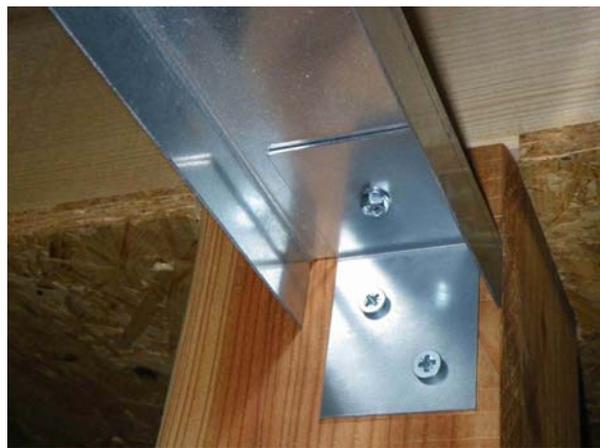
Figure 6-5: Mounting the end profile
