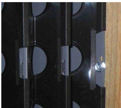
Figure 6-27: Fastening to the wooden post
