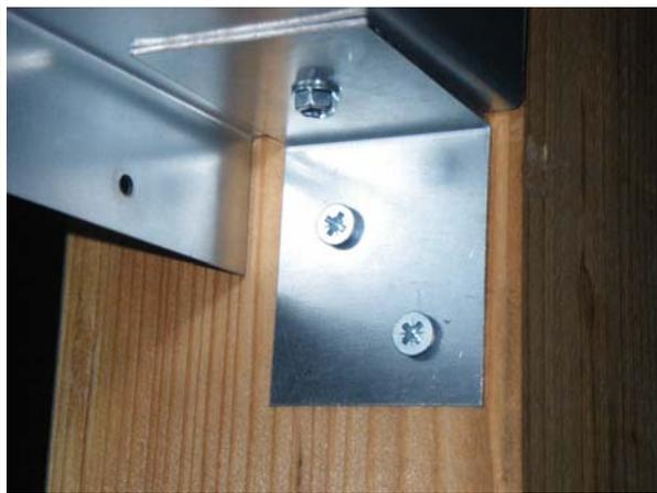
Figure 6-4: Mounting the fixing profile
