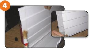
4. Apply the Tangit adhesive **immediately** to the glued joints on the inside and outside of the drip trough using the brush. Observe the time for which Tangit adhesive containers may be open (4 minutes at 20 °C).
