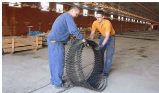
Figure 6-4: Uncoil the auger
